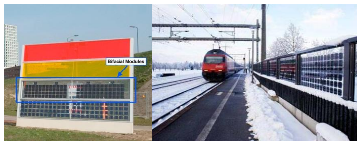
Fig. 26 Applications of vertical bPV modules as noise barriers (Switzerland, 1997).
