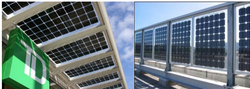
Fig. 25 The applications of bPV modules in BIPV.
